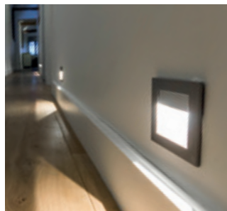
Low-level wall lighting
