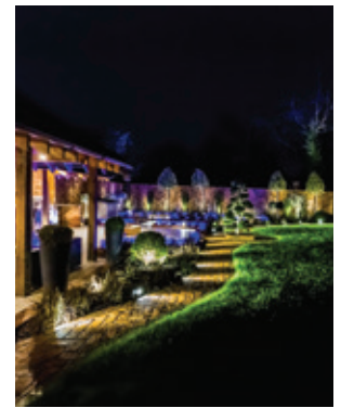
Light spread across installation
